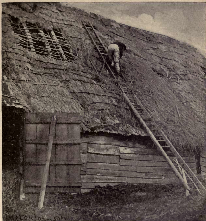
Patching the Thatch Roof of a Barn
